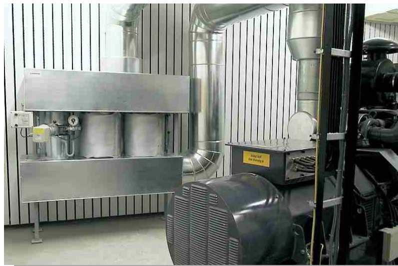
Soot particulate filter CRP-N2, for power systems up to 300 kVA with bypass, pressure monitoring, and control panel
